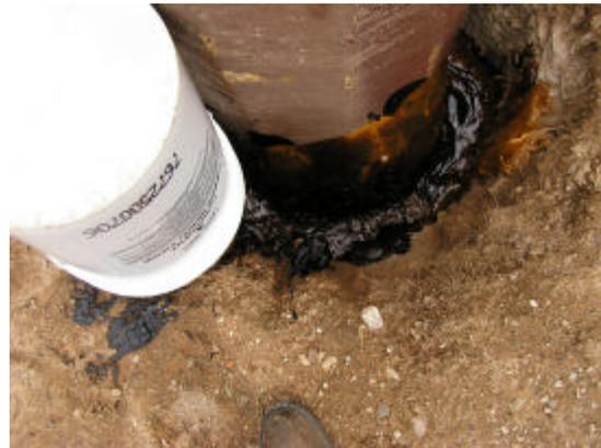
Photo Showing Poly-Set Being Poured Into Hole
