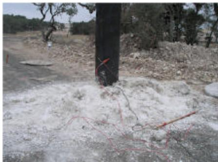
*Photo showing pole set with native spoils with megger wires attached to ground rod.*
