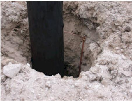
*Close up of hole. Notice the location of the ground rod in the annular space*
