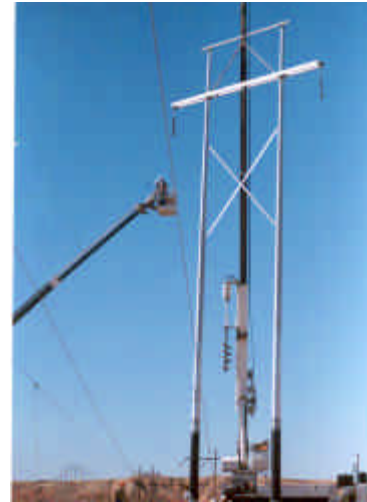
H-Frame being set into position
