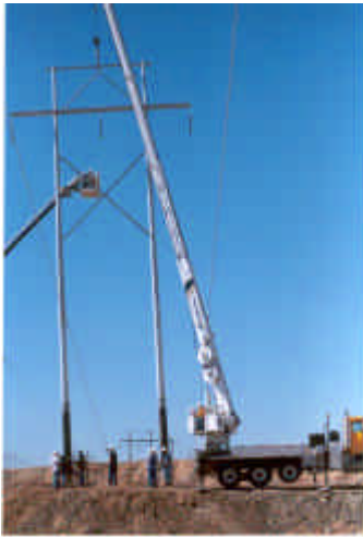
Pole being lifted into position
