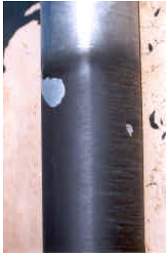
Pole showing Corro-Coat issues
