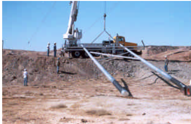
H-Frame on the ground being lifted
