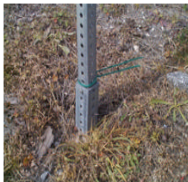
Perforated Square Metal Tubing (Driven or Augered)
