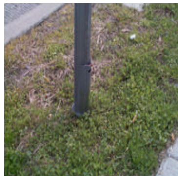
Wedge Anchor Thin Thin Wall Tubing (Driven or Augered)
